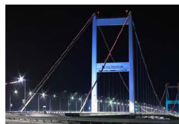
Irtys River Bridge, Kazakstan
