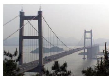
Humen Bridge, Hong Kong, China
