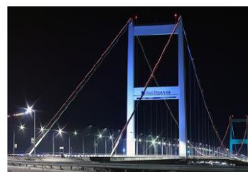
Irtys River Bridge, Kazakstan
